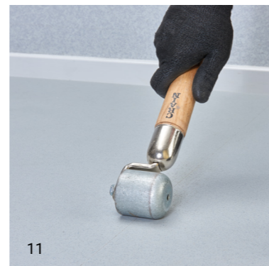
11 A hand roller or heavy roller can be used at all seams/perimeter immediately after installing to ensure sufficient contact has been made.
