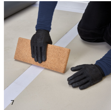
7 To ensure the QuickLay tape is firmly positioned correctly, simply press down with a hand roller or cork board.
