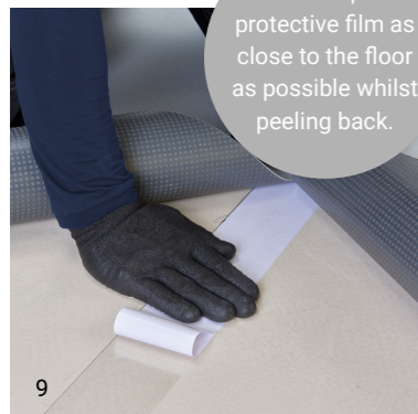
9 Carefully peel away the protective film from all areas where the tape has been applied.
