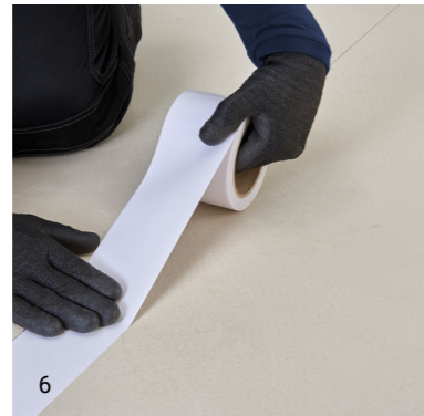
6 Apply the QuickLay double-sided tape along the marked seams.
