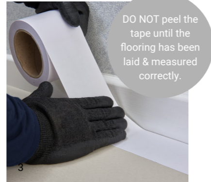
3 Apply the QuickLay double-sided tape around the perimeter of the room and at any doorways, set 2mm away from the edge of the room.
