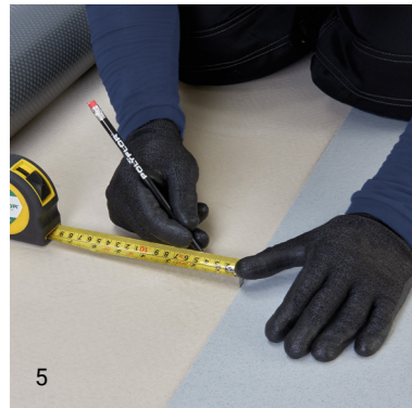
5 Measure 37.5mm away from the side of the seam and mark with a straight edge or chalk line.
